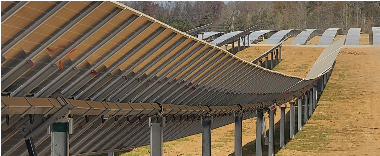
Figure 2: Genius Tracker TF tables following site undulations.
