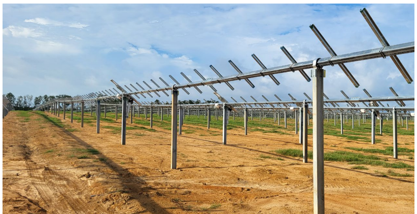
Figure 1: Straight-tube trackers requiring grading and additional pile reveal to account for site terrain.
